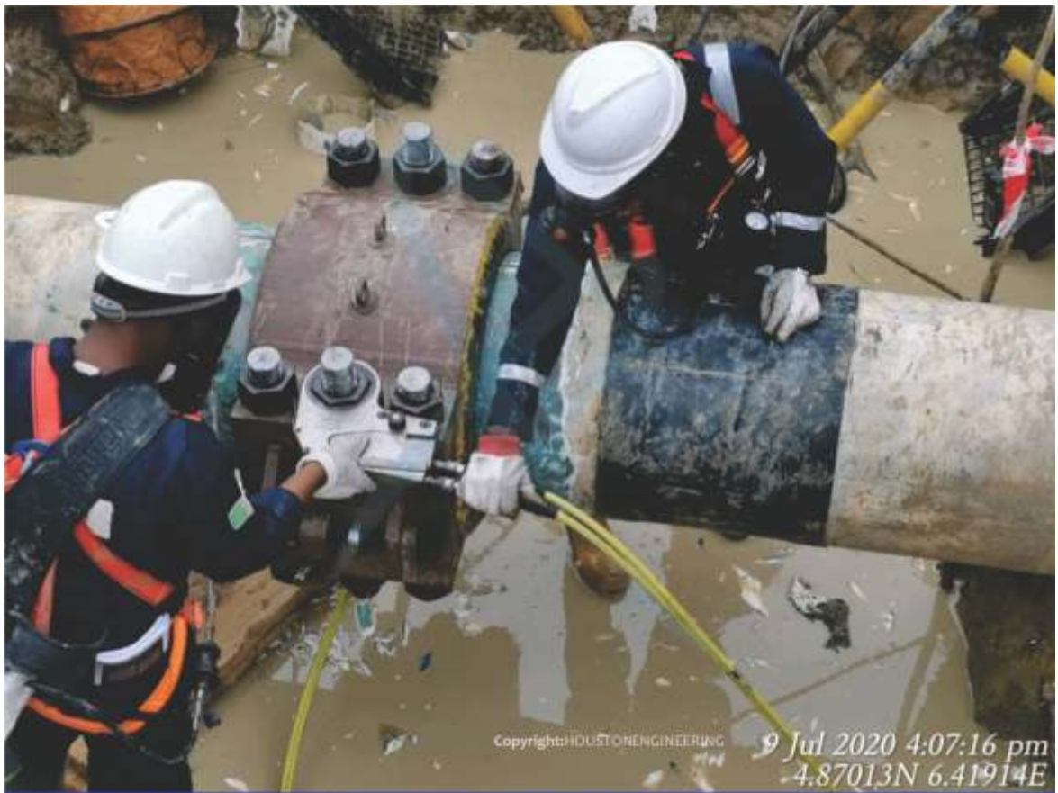
PNEUMATIC TORQUEING OF 20" CLAMP ON 20" KOLO CREEK - SOKU PIPELINE
