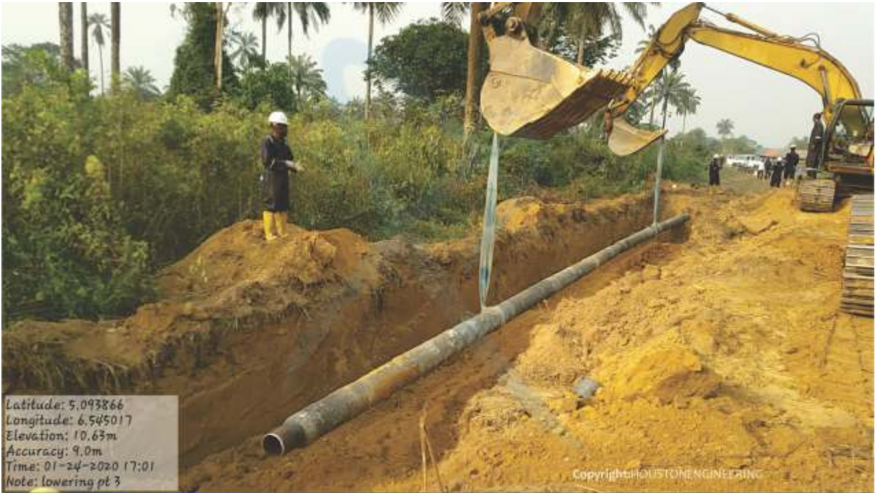
LIFTING AND POSITIONING OF THE REPLACEMENT PIPE ON 8" UBIE PIPELINE
