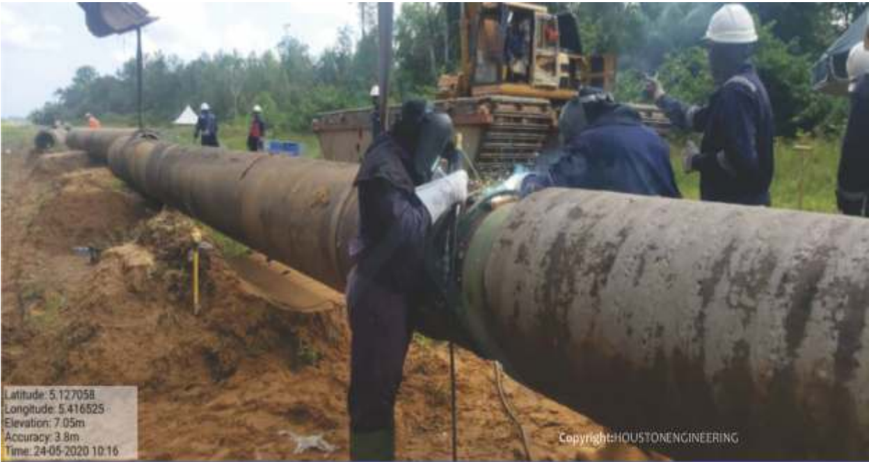
SMAW WELDING PROCESS ON 24" TRP RIVER CROSSING
