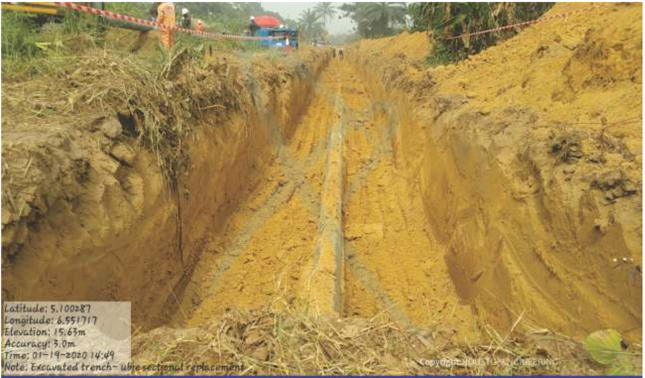
EXCAVATION TO EXPOSE DEFECT POINT ON 8" UBIE PIPELINE
