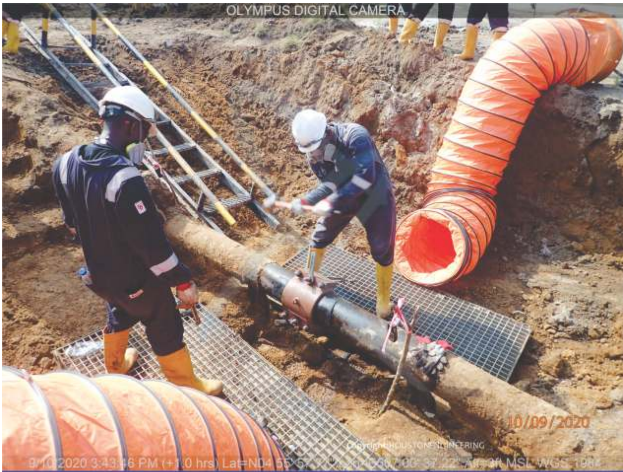
LEAK REPAIR BY CLAMPING ON 8"DL AGBADA2 - NKPOKU
