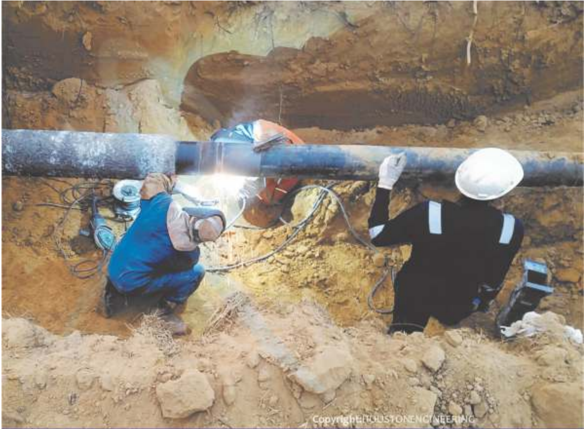
SMAW WELDING PROCESS ON 14" OKORDIA - RUMUEKPE PIPELINE
