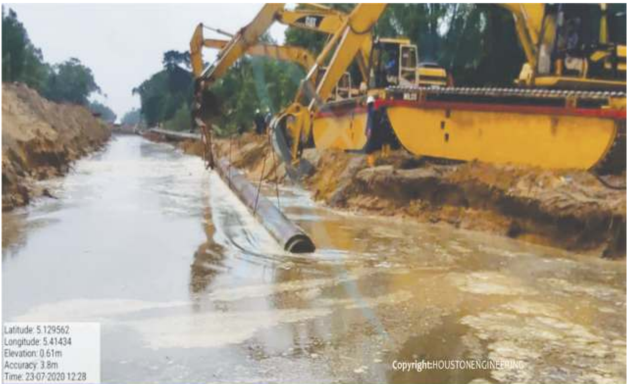
LOWERING OF REPLACEMENT FOR 24" TRP PIPELINE KP29
