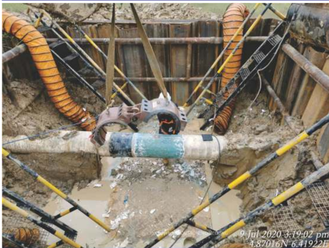
INSTALLATION OF 20" KOLO CREEK - SOKU PIPELINE
