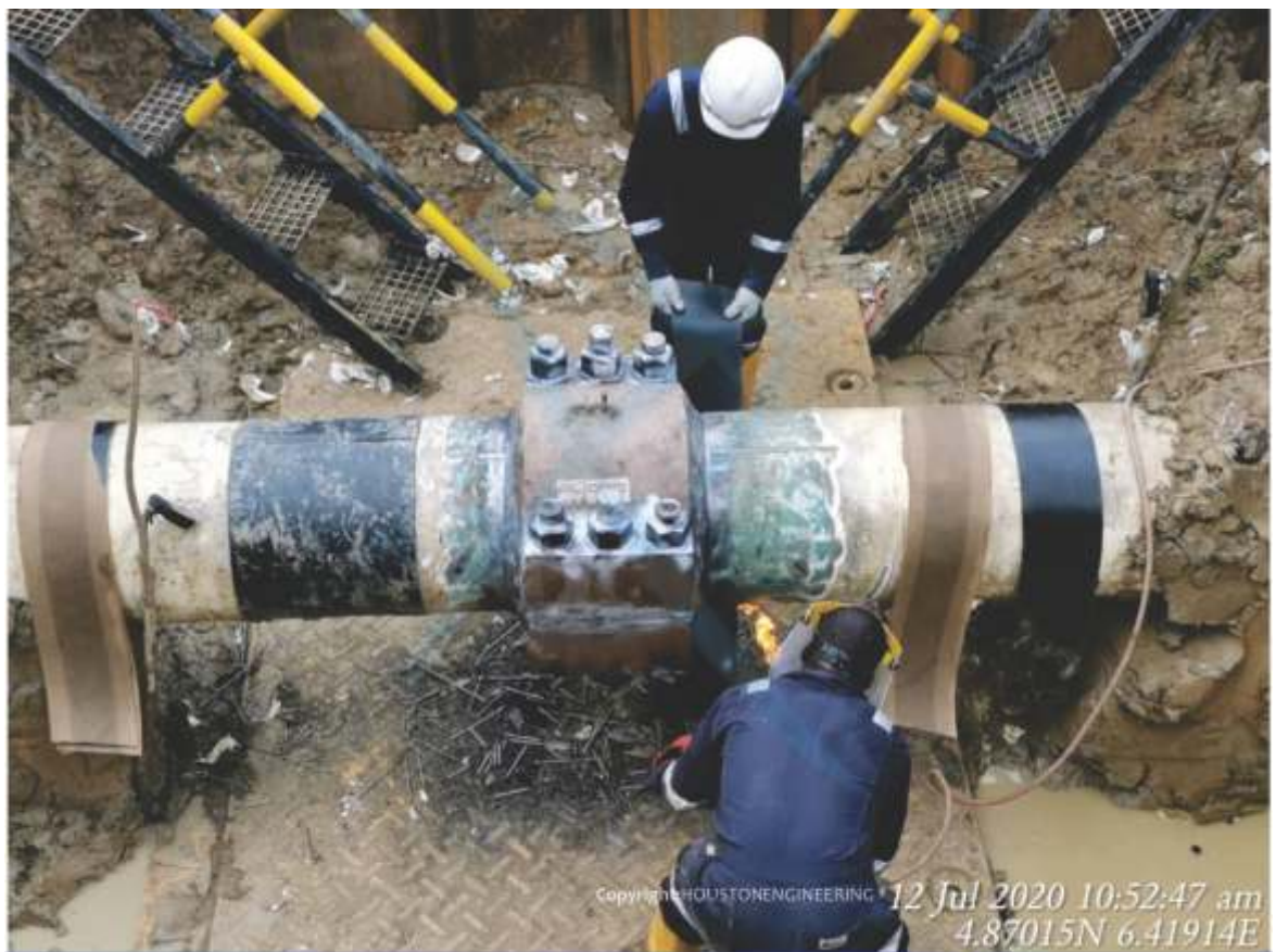
PIPE COATING ON 20" KOLO CREEK - SOKU PIPELINE
