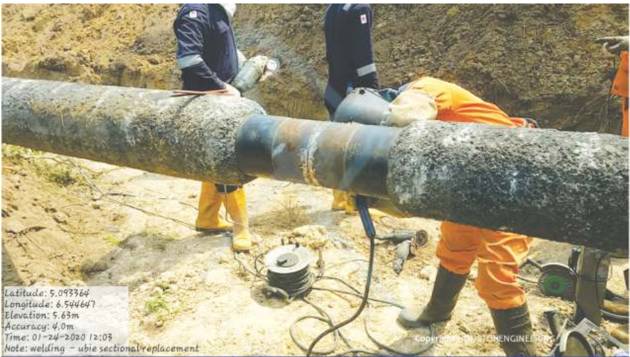
SMAW WELDING PROCESS
