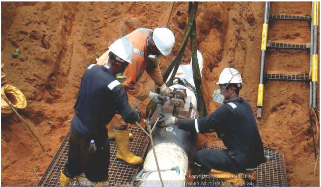
CLAMP INSTALLATION ON 18" ASSA - RUMUEKPE PIPELINE
