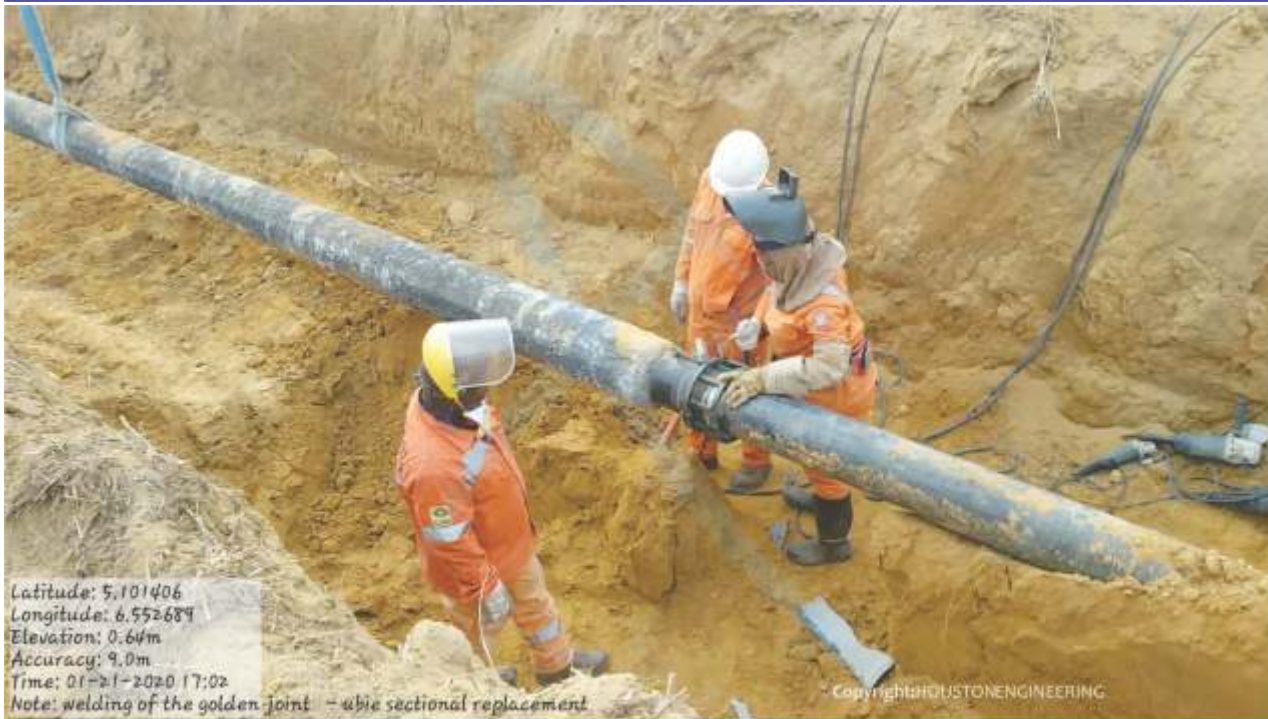
FIT UP ON 8" UBIE PIPELINE
