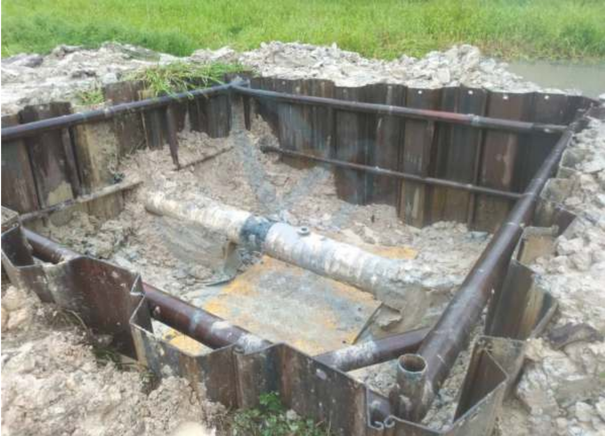
COMPLETED CLAMP WELDING ON 20" KOLO CREEK - SOKU PIPELINE
